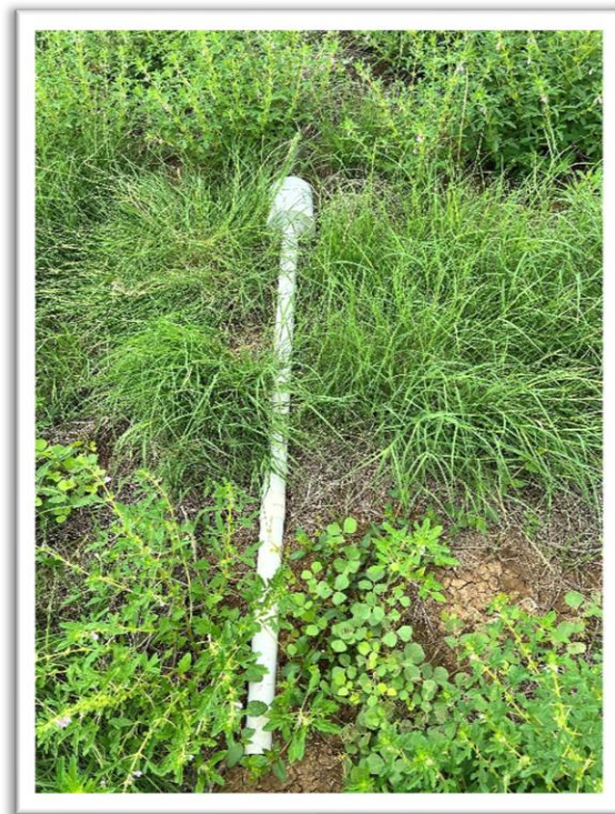
Figure 14 - DDG2 knocked over (15 April 2024)
