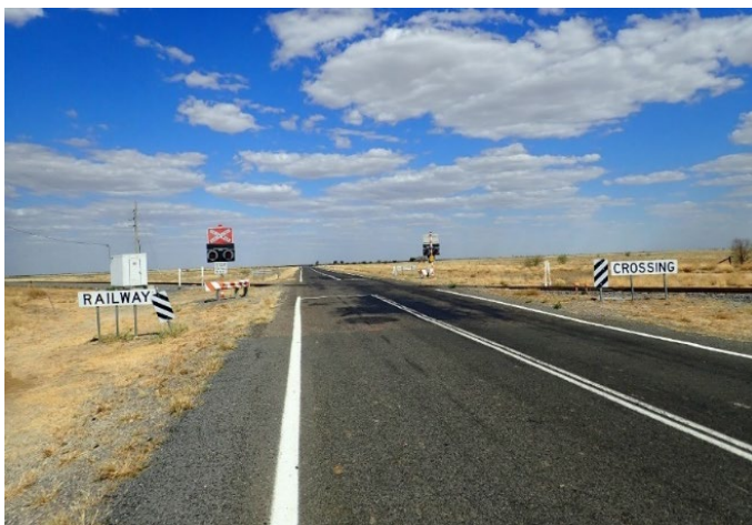
Figure 1: Existing Railway Crossing Flinders Highway (east facing)
